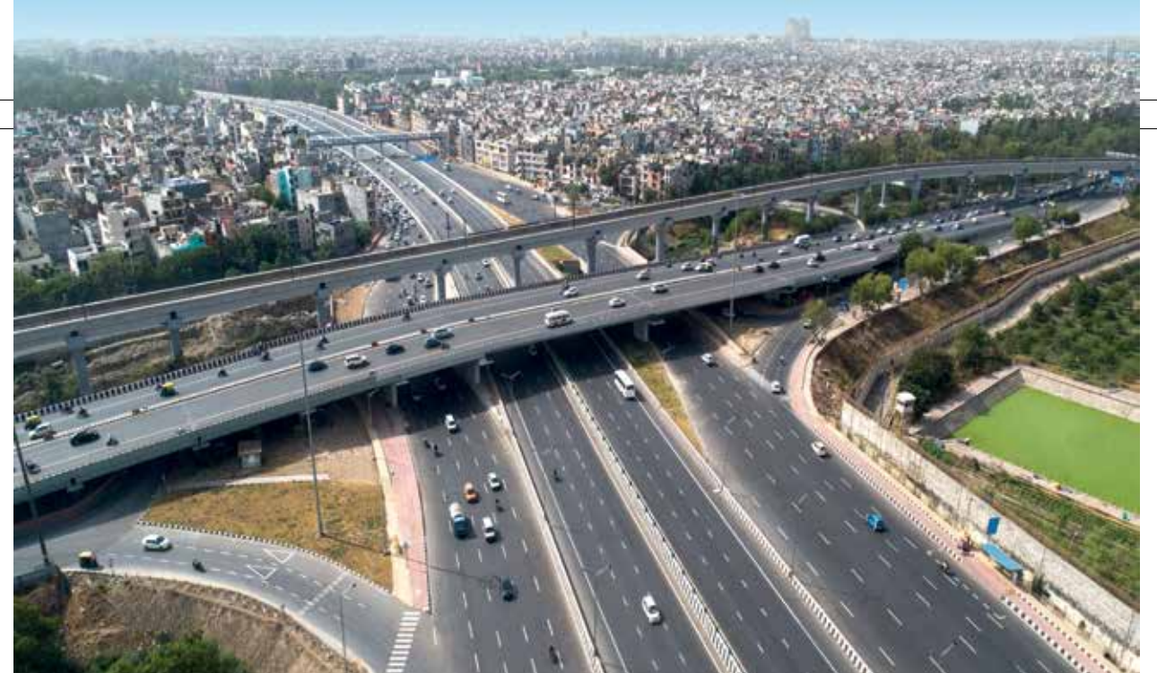
▲ Perhaps no other agency has worked at such breakneck speed to give the country its much-needed infrastructure.
