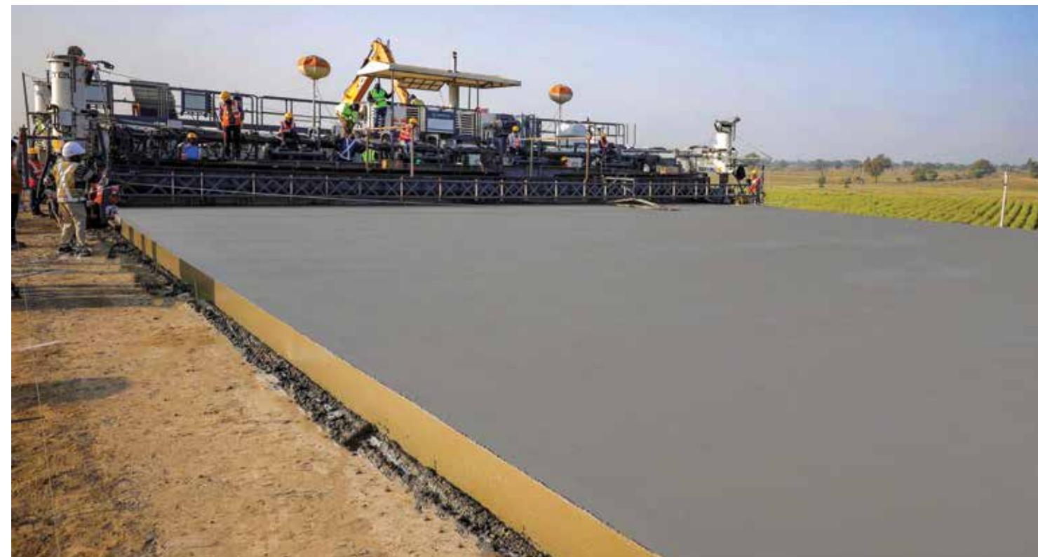
▲ The Wirtgen SP 1600slipform paver that created the world record.
